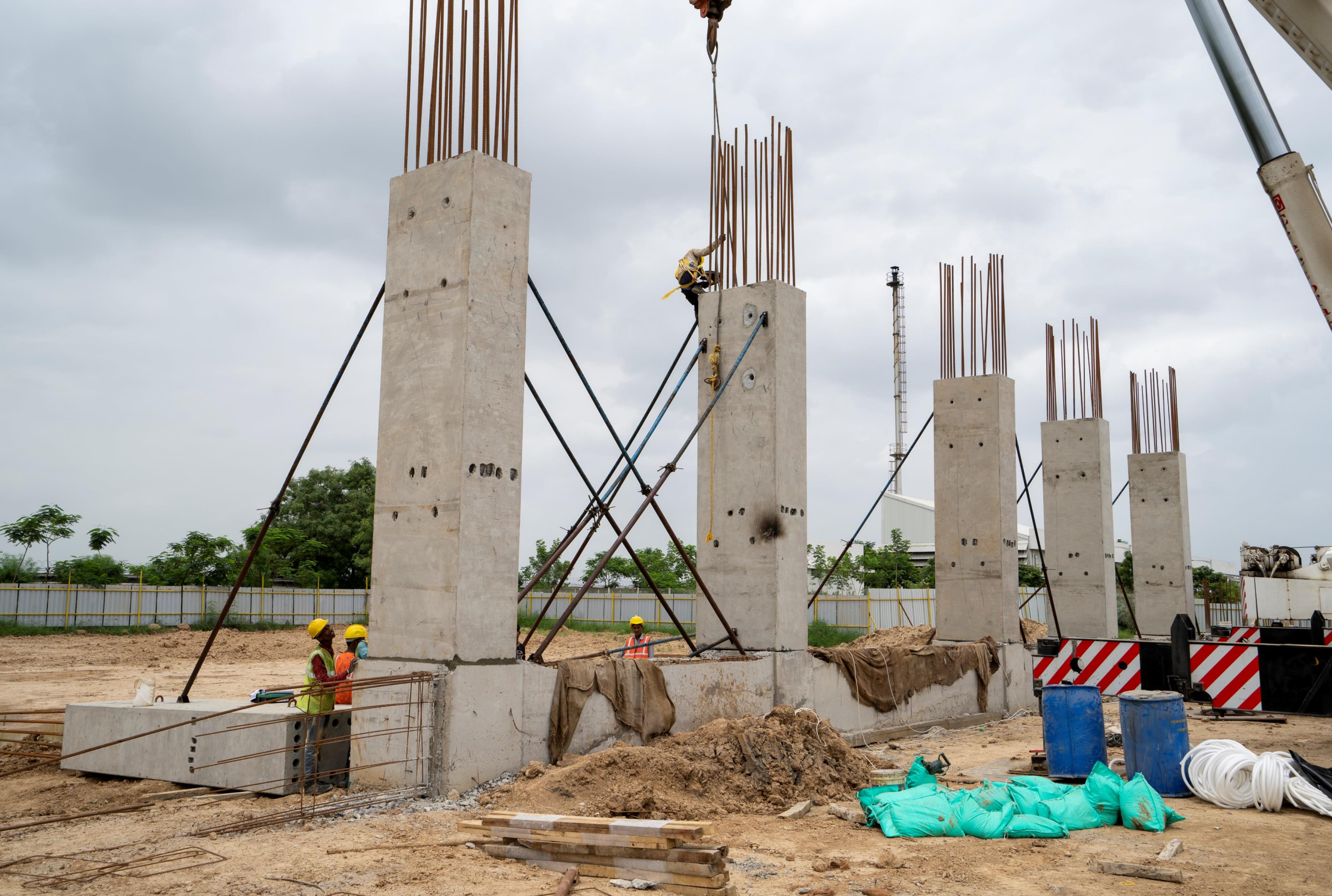
Erection of Column
